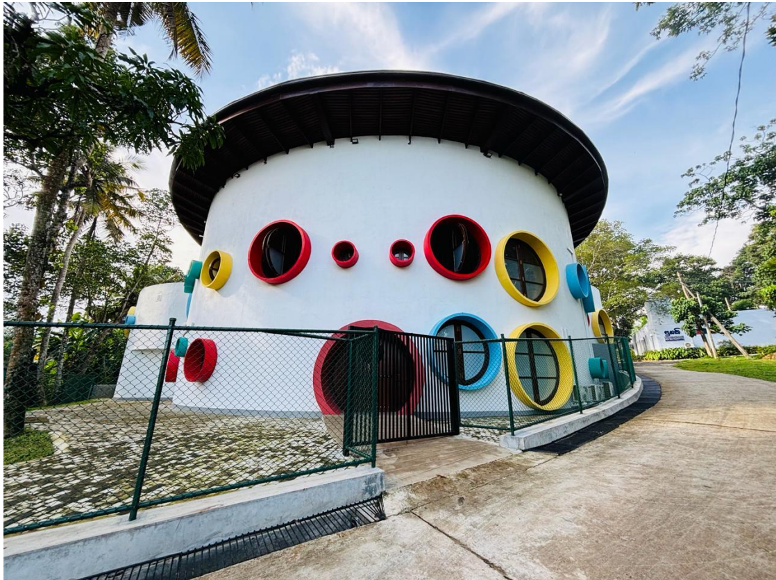
Figure A.2: Pragathi Child Intervention Centre exterior.
